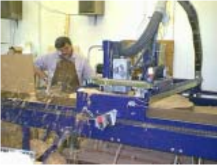
Leveling the slabs
